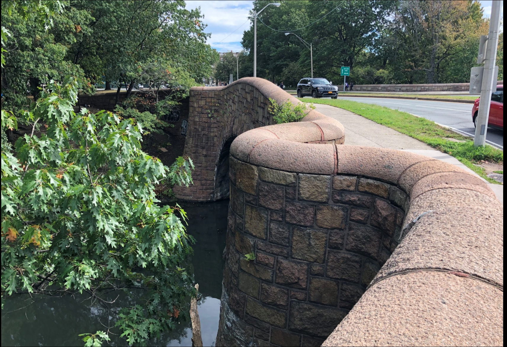
Stone bridge by HH Richardson.
