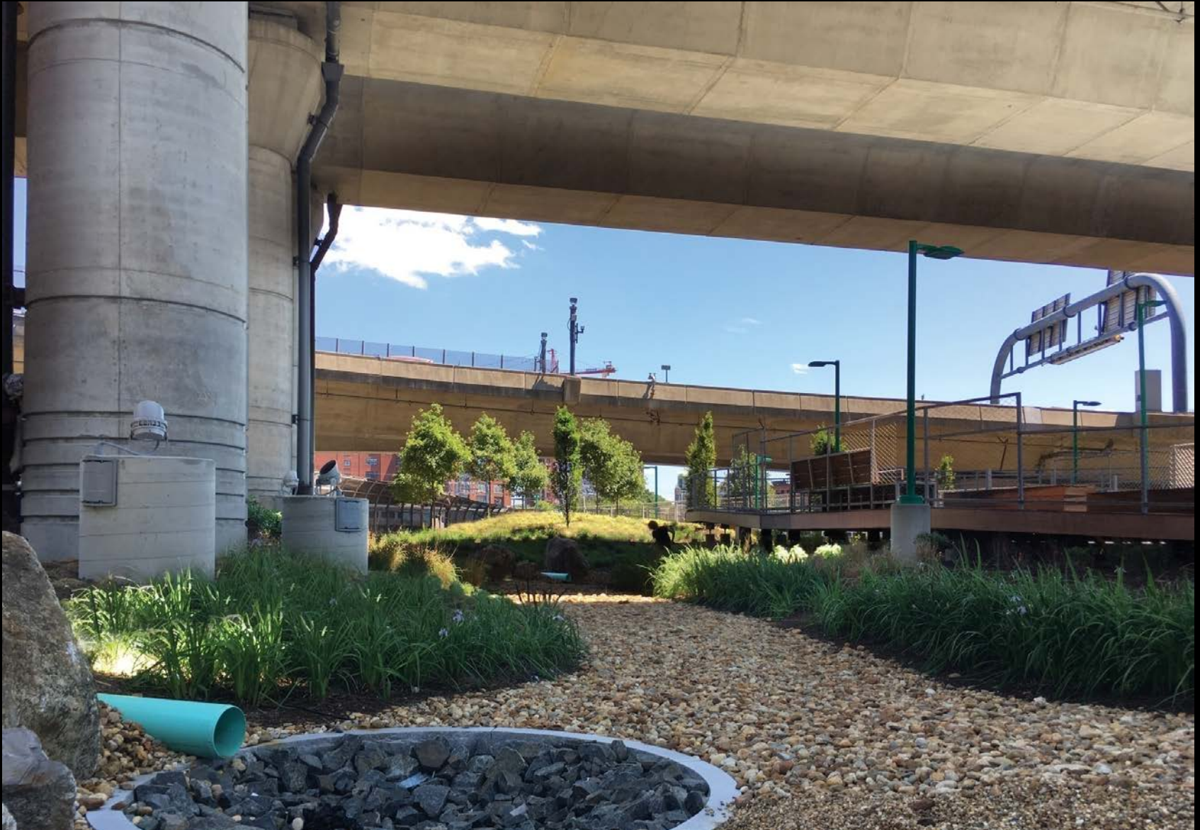
Stone filled 'dissipation basins' distribute runoff into the filtration and retention landscape
