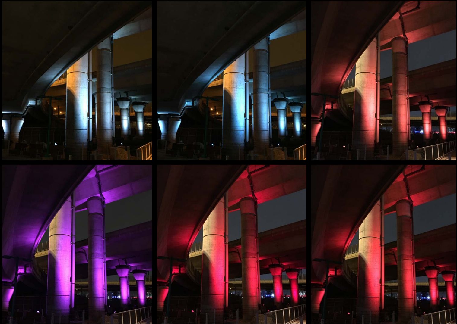
Commissioned up lighting at Underground at Ink Block
