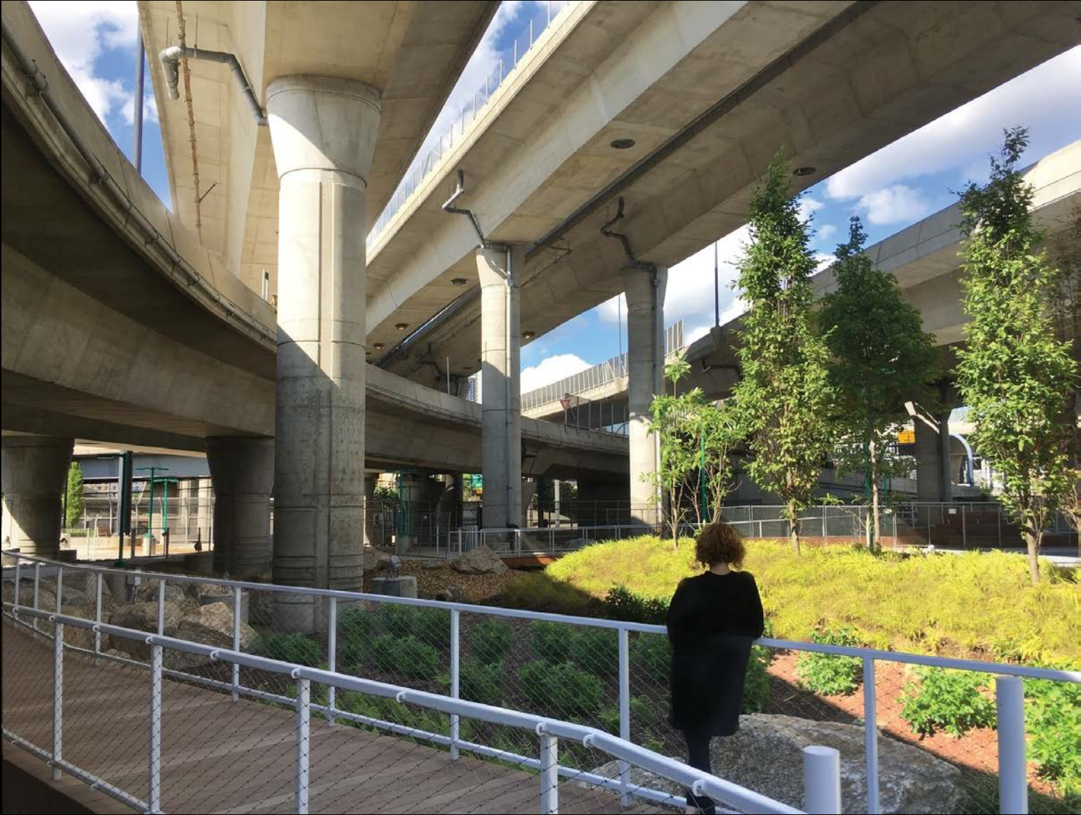
Daylight through the viaduct
