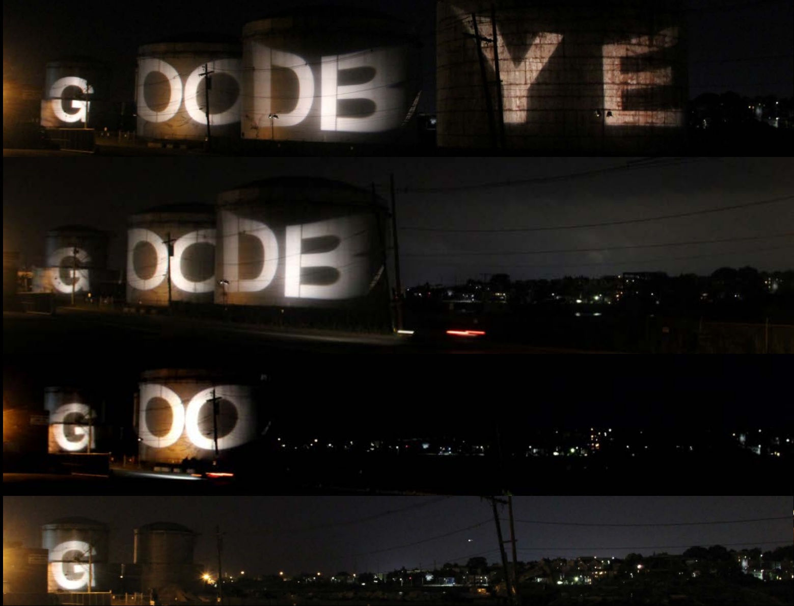
Temporary light projections on the Coastal Oil tanks along Chelsea Creek during demolition. Letters disappeared as tanks were demolished over 1 month.
