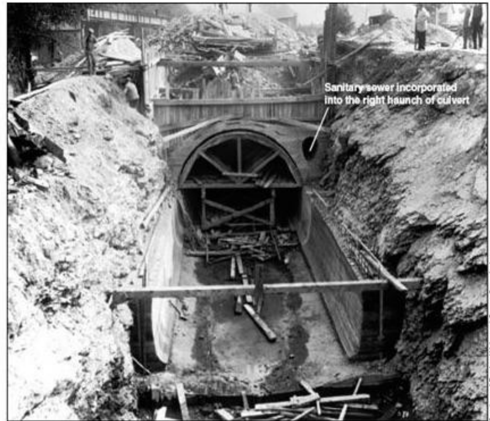
Figure 11. The culverting of Stony Brook at Forest Hills, about 1905.
