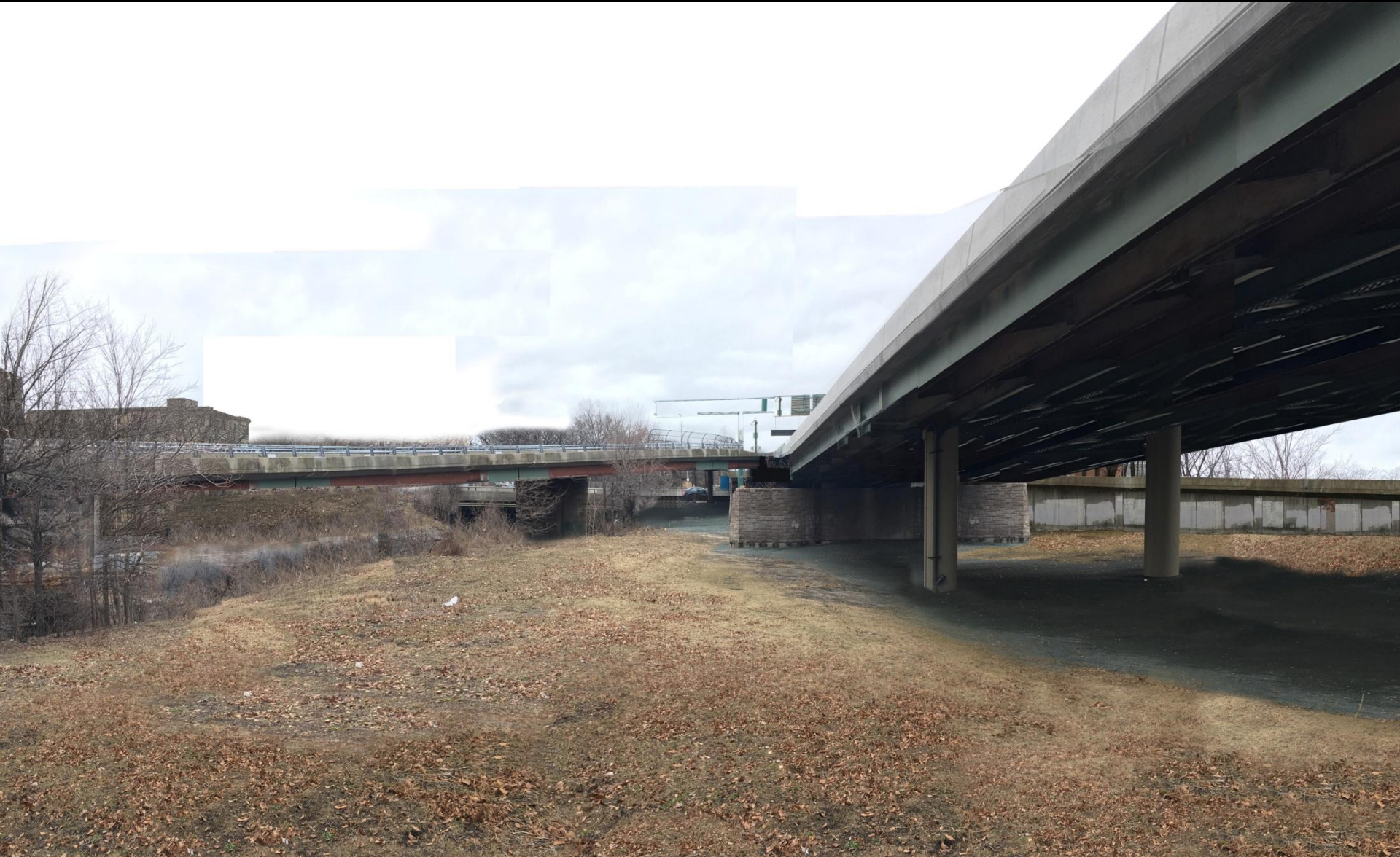
Existing: from Commonwealth Ave looking south
