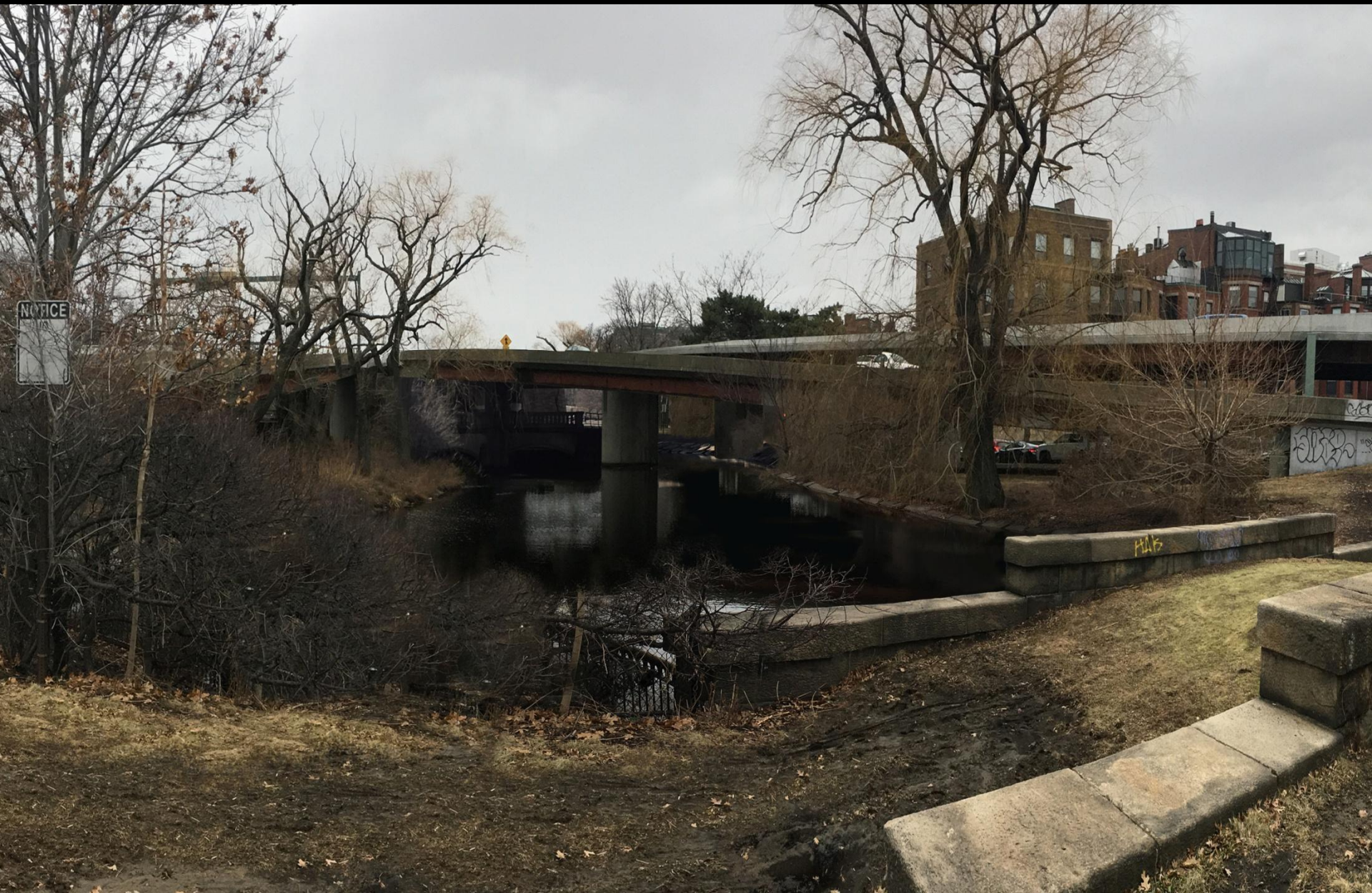
Existing: looking south from Storror EB ramp area
